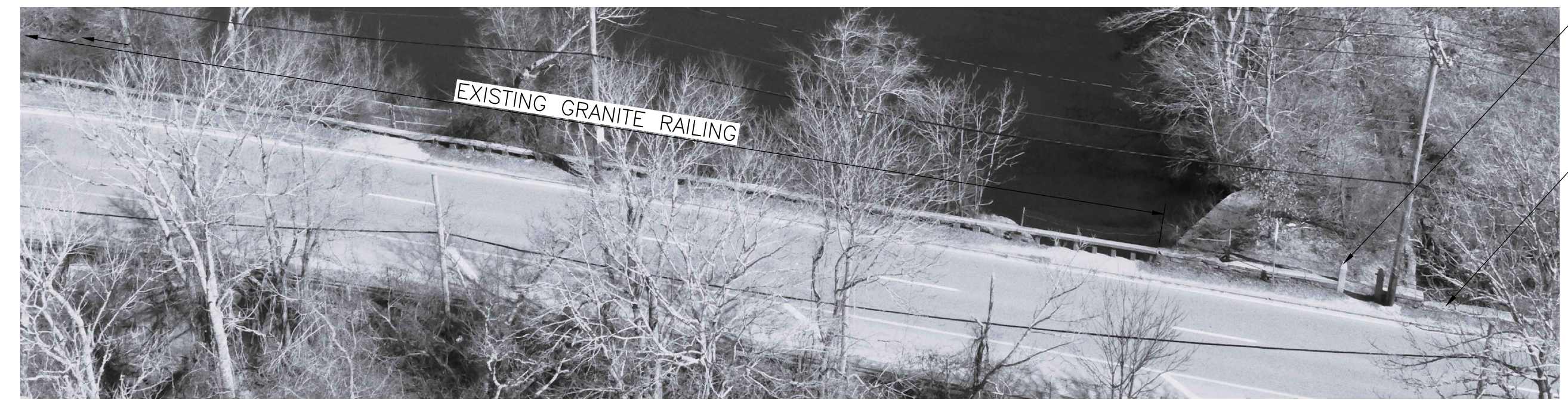
AERIAL VIEW OF EXISTING GRANITE RAILING AND PIERS NOT TO SCALE
